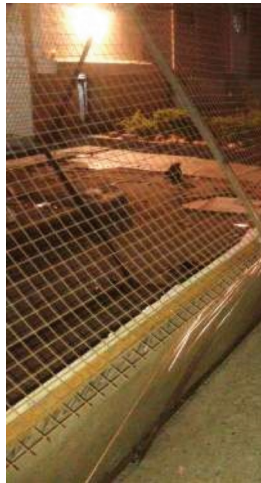
Fig. 15. Primary structure, welded with meshed-steel sheet – module 1729
