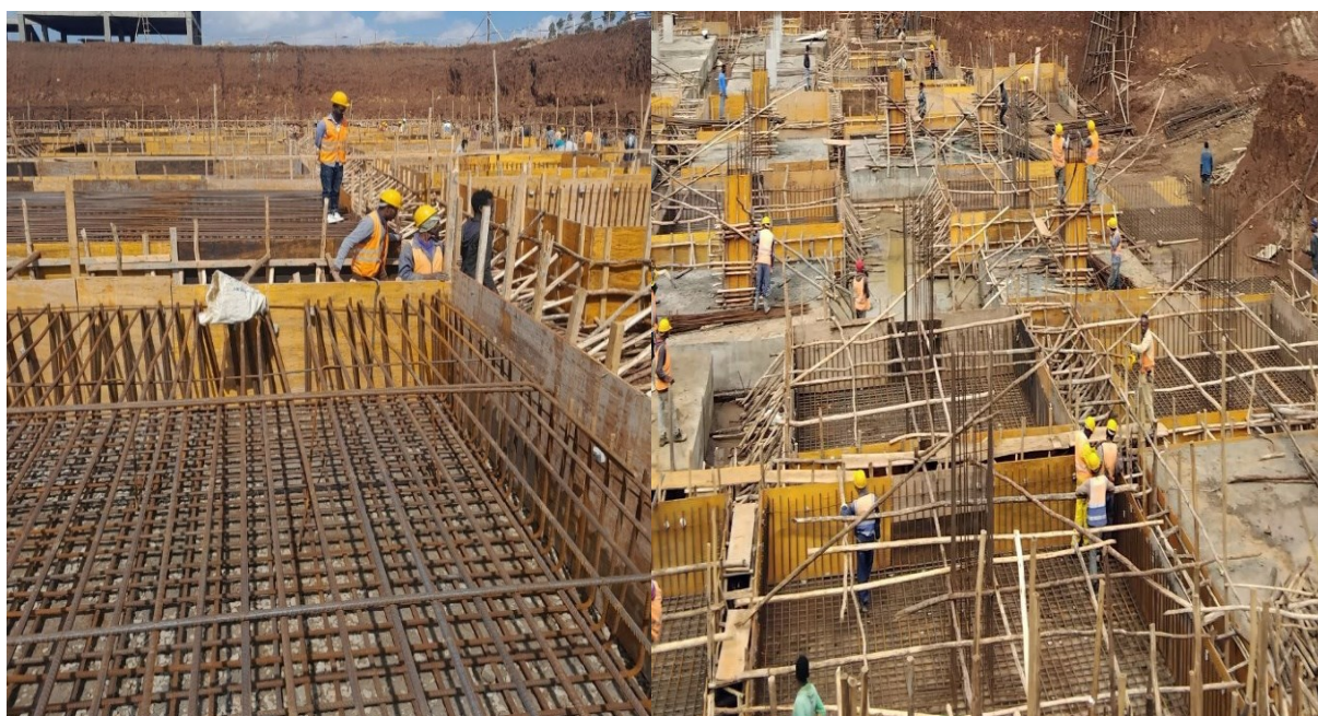
Figure 2.14 Rebar Placement for Isolated and Combined Footings Spaced by 5cm from the formwork.
