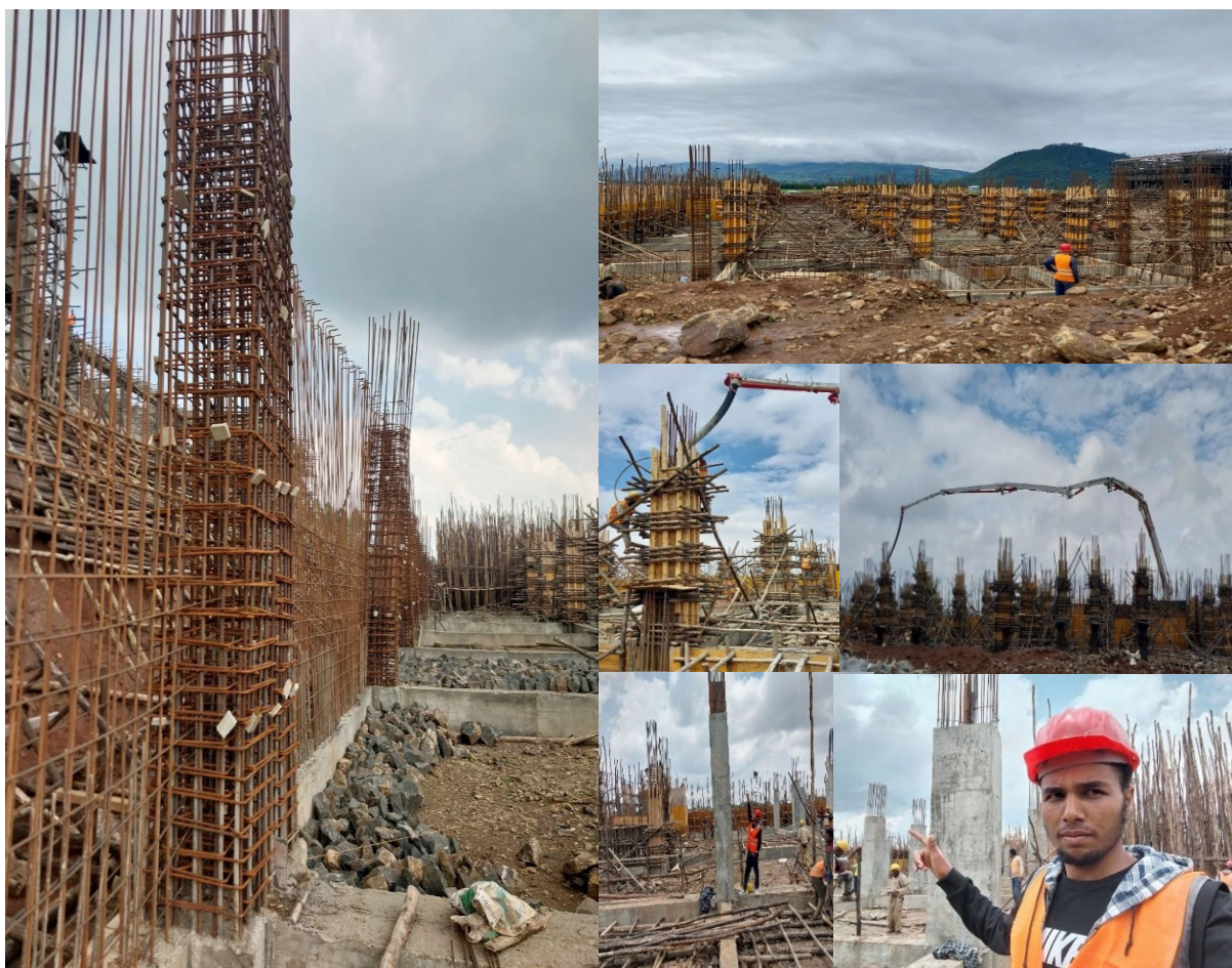
Figure 2.29 Basement Column Preparation, Formwork, and Concrete Pouring and executed column.
