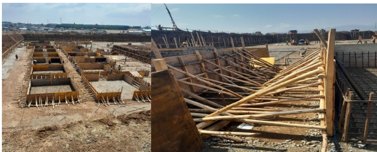
Figure 2.13 Footing Formwork of MHB with 50 mm Cover.
