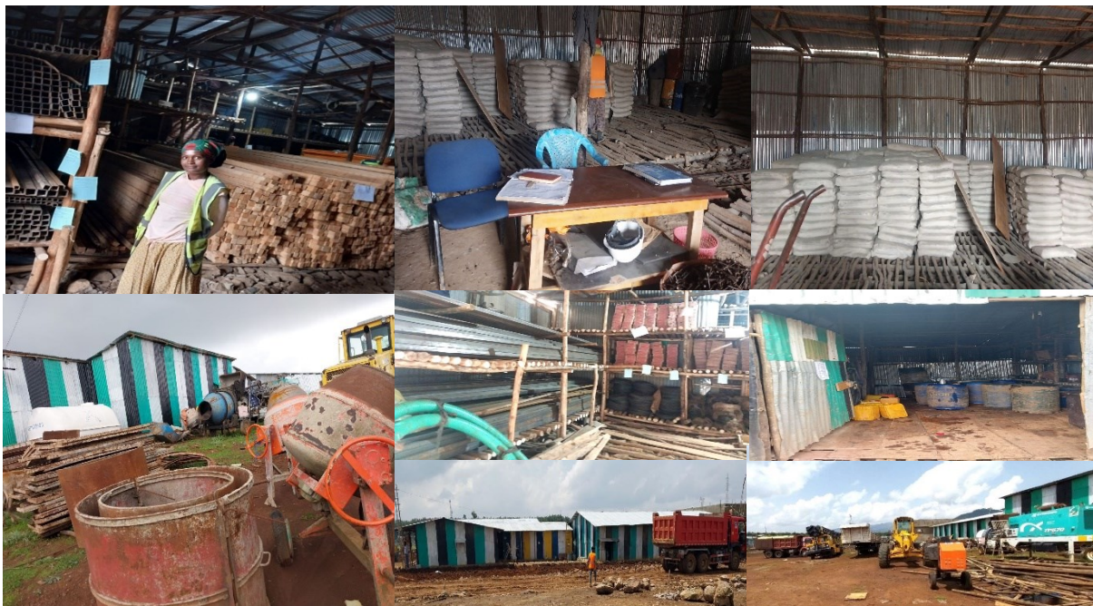
Figure 2.49 Material Storage and Stalking on the site.
