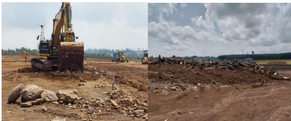
Figure 2.11 Site Clearance and Grubbing Activities of the project.
