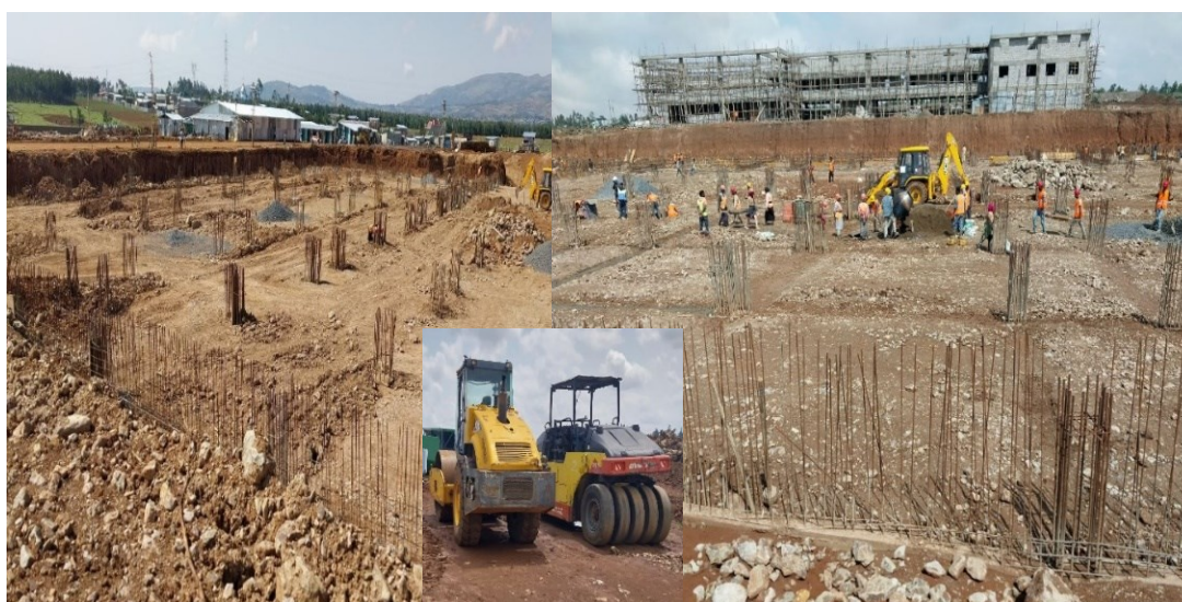
Figure 2.16 Backfill Compaction of MHB to Achieve Maximum Dry Density.
