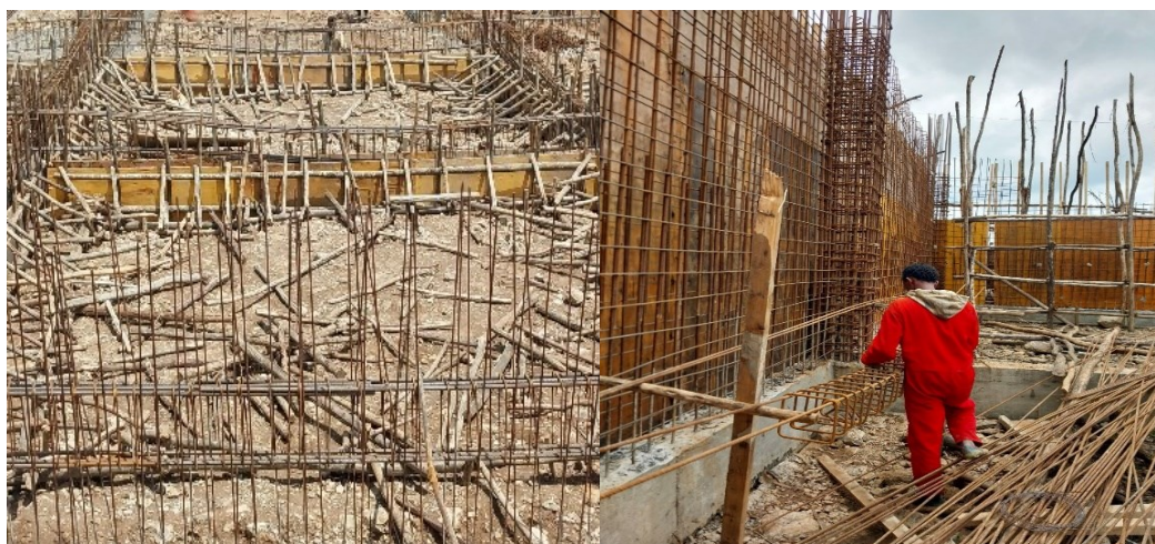
Figure 2.33 Retaining Wall Reinforcement installation and formwork erection.
