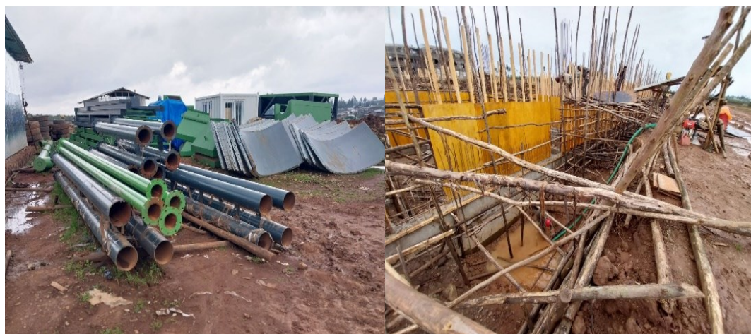
Figure 2.41 OCTG Pipes and Pump Removing Accumulated Water.
