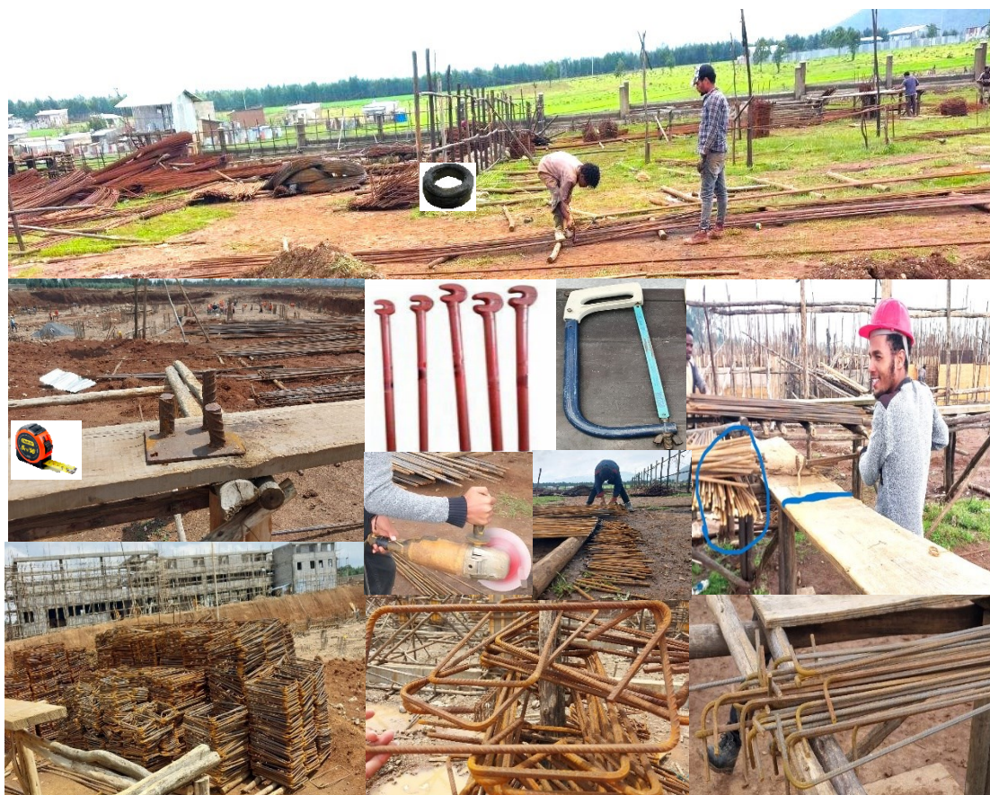
Figure 2.42 Bar Storage, Cutting, and Bending Area on Site.
