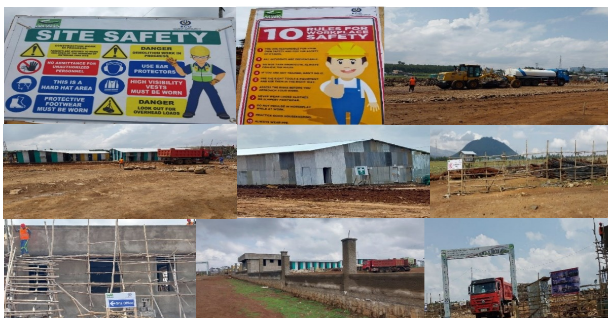
Figure 2.9 Site Layout before Mobilization, showing key facilities (i.e. Site Offices) and safety signage.
