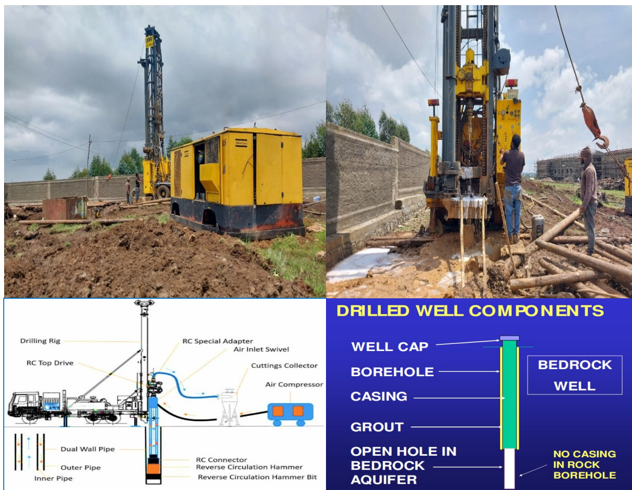
Figure 2.46 Drilling operation of a borehole to access underground water for the Project.
