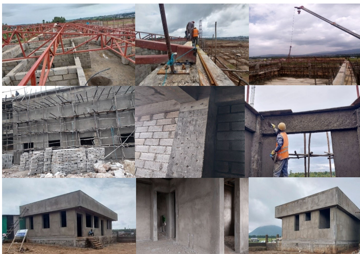
Figure 2.44 Finishing Work of Administration and Pharmacy Buildings.
