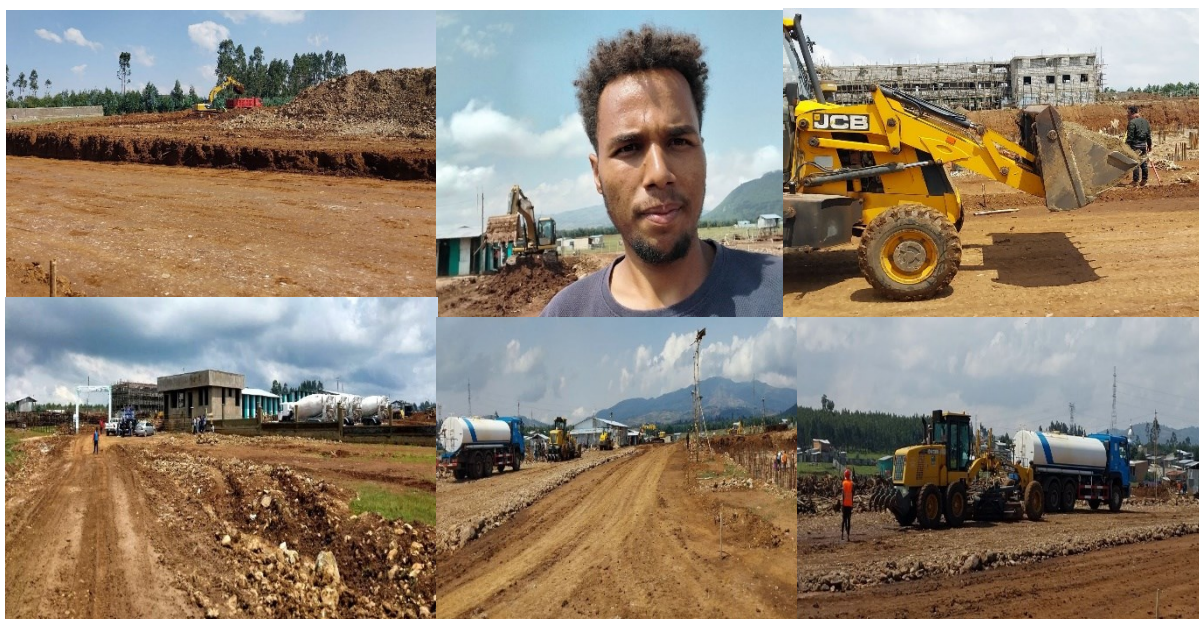
Figure 2.47 Expansive Soil Removal and Asphalt Road Layering of the project.
