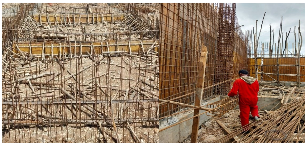
Figure 2.33 Retaining Wall Reinforcement installation and formwork erection.
