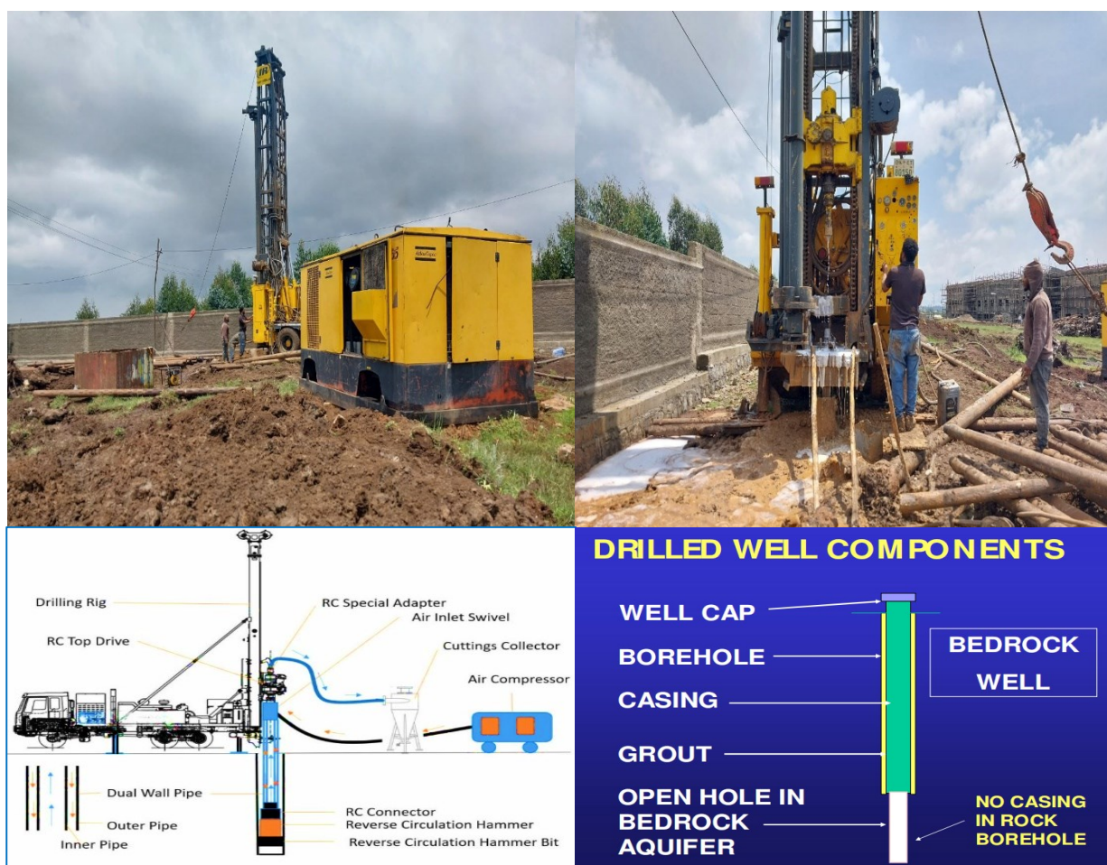
Figure 2.46 Drilling operation of a borehole to access underground water for the Project.
