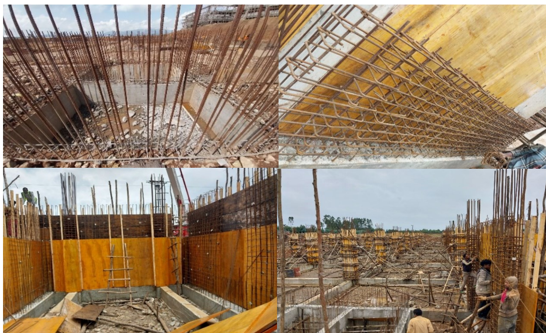
Figure 2.36 Shear Wall reinforcement installation formwork constructing
