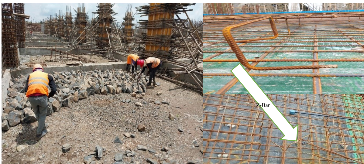
Figure 2.39 Crushed Stone Sub-Base for Basement Slab of MHB.
