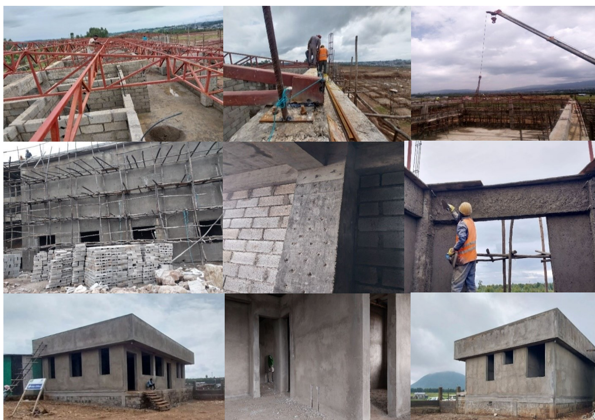
Figure 2.44 Finishing Work of Administration and Pharmacy Buildings.
