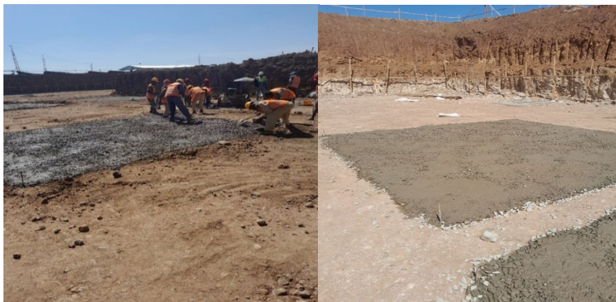
Figure 2.12 Lean Concrete Mixing using a Drum Batch Mixer and Placement under MHB Footings.
