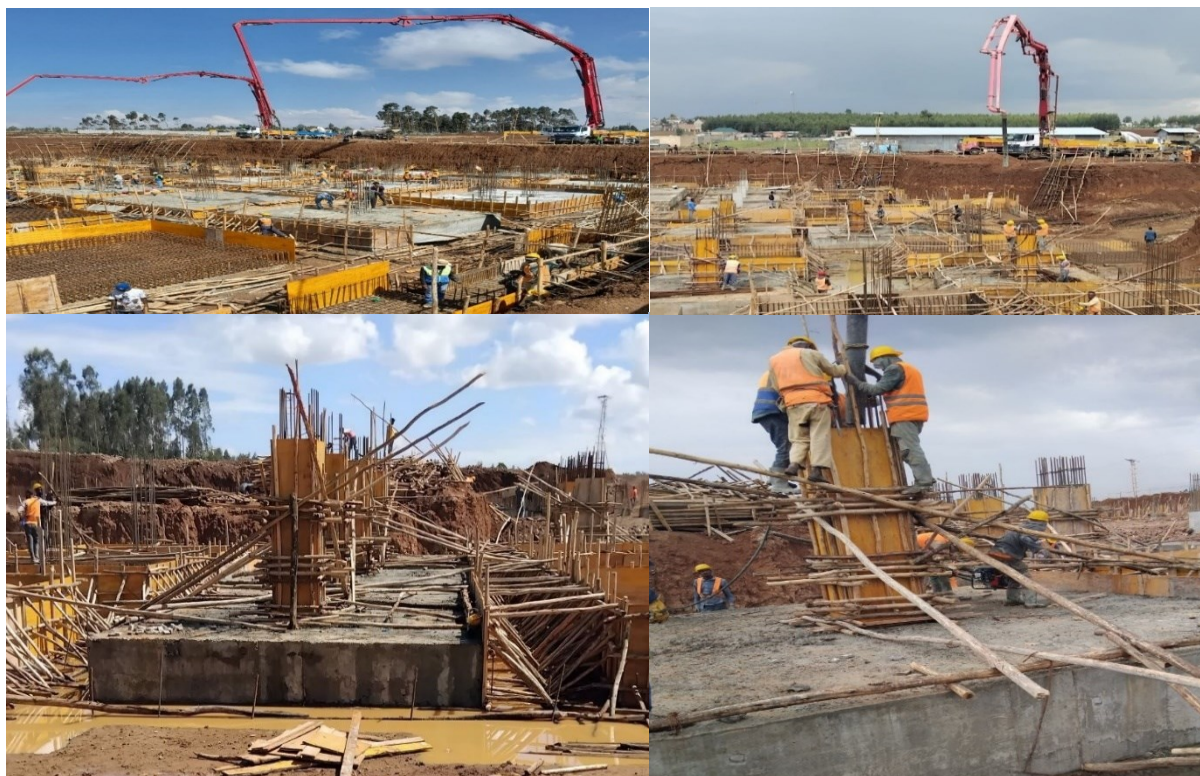
Figure 2.15 Placement of Concrete for Footing Pads and Column Starters via Pump Truck.
