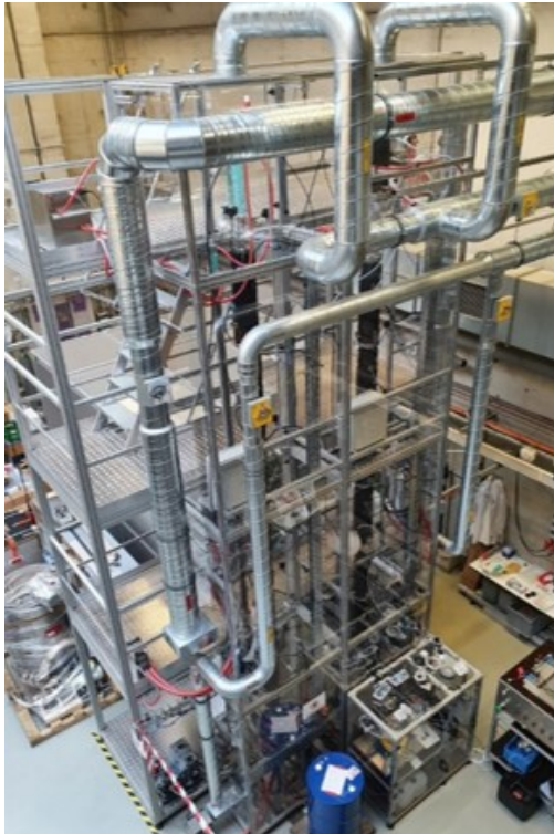
(a) Continuous distillation mini-plant.
