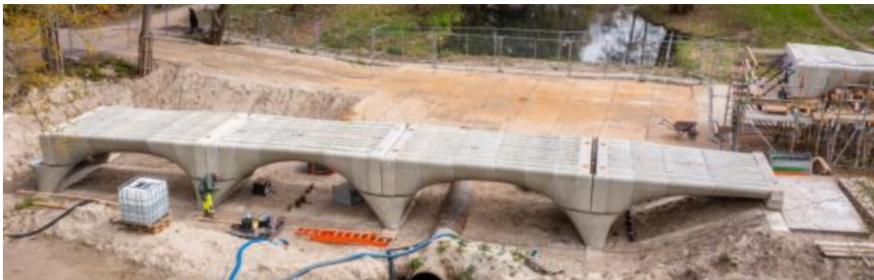
Figure 9: Assembly of the final bridge on location [25].
