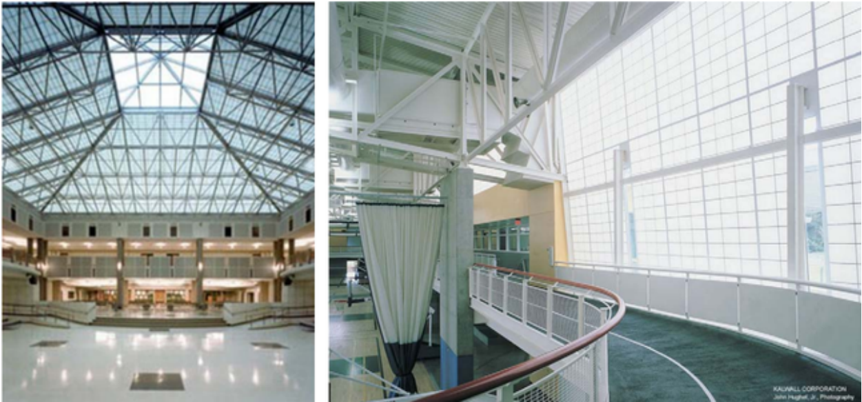
Figure 3: Two examples of translucent aerogel insulation as a thermal insulation solution for daylighting [3].
