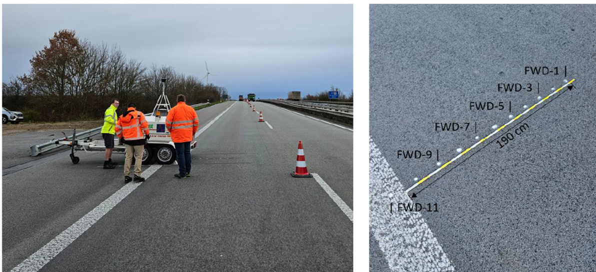
Figure 16: Positioning of the FWD perpendicular to the direction of travel
