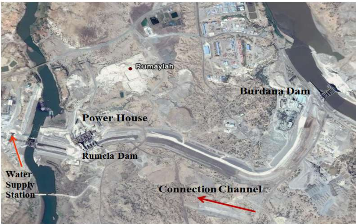
Fig (8c) Rumela, Burdana Reservoirs and the Linking Channel
