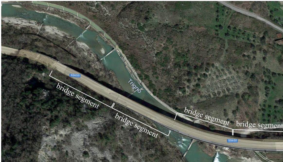
Figure 5.11: The Trigno V bridge over the Trigno river that carries SS650 north of Trivento, Italy, is made up of seven repeating concrete bridge deck b .
