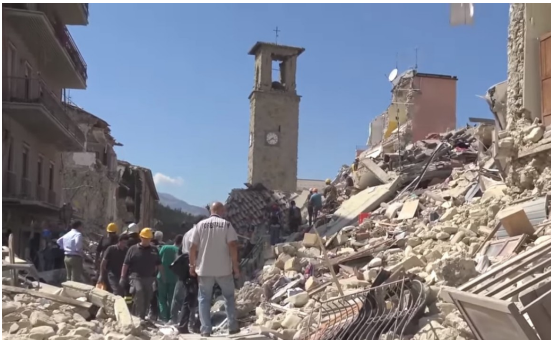
Figure 3.22: The town center of Amatrice, Italy, after the August 24 th 2016 earthquake that measured 6.2 on the moment magnitude scale; note that the bell tower (lower natural frequency) is still standing while shorter stiffer structures (higher natural frequency) have suffered extensive damage. a
