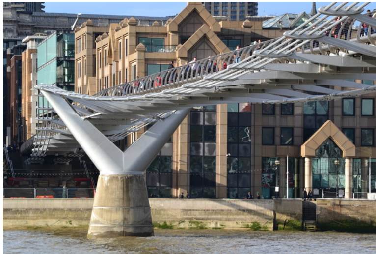
Figure 3.11: View of Millennium Bridge in London UK a .
