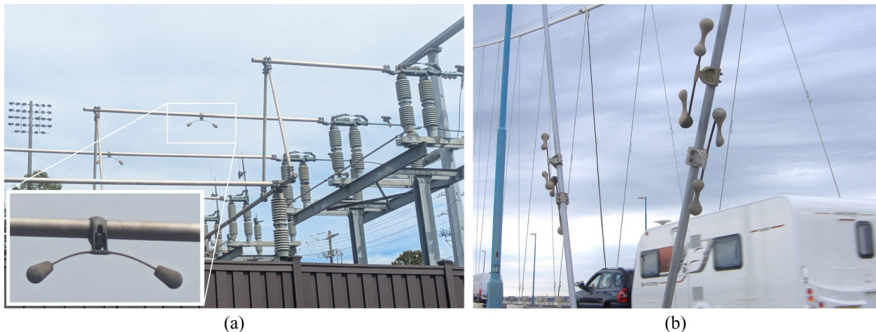
Figure 6.4: Vibration absorbers deployed on wind excited cables showing: (a) a Stockbridge damper mounted on a rigid bus conductor in an electrical substation, and; (b) a dogbone damper on a suspender cable of a suspension bridge a .
