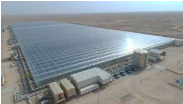
Figure 5: Aerial Photo of the Miraah Commercial Project (© GlassPoint, Reproduced With Permission).
