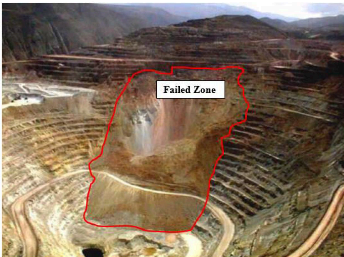
Figure 1: A porphyry copper mine in South America suffered a major slope failure. [21]
