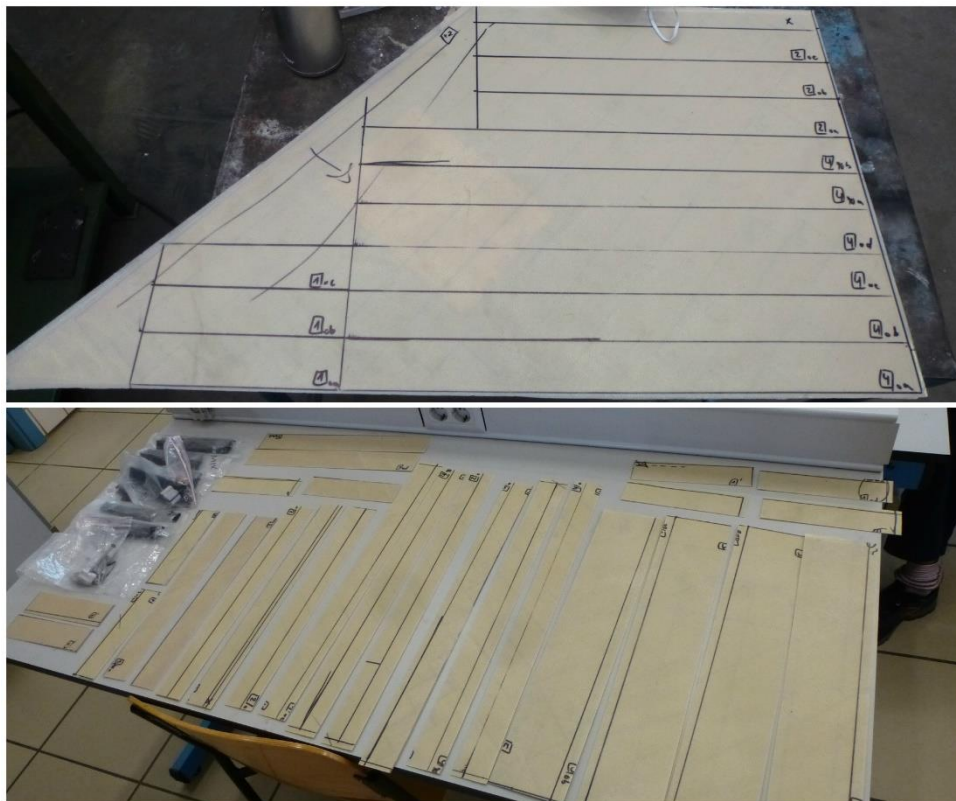
Figure A-6. Above : Fiberglass panel ready to be cut; Below : All tabs already cut.
