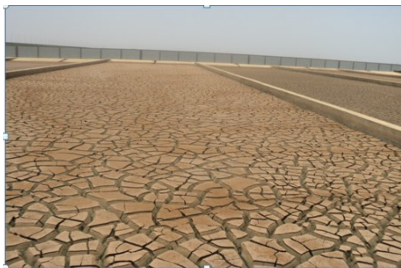
Plate 3: Drying of the sludge in large ponds
