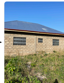
Single-story building with columns using oyster shell concrete
