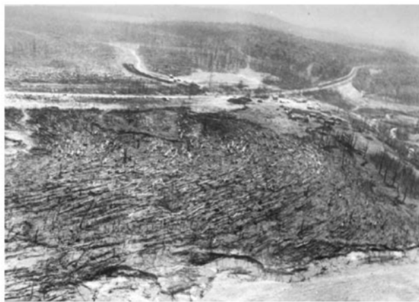
Figure-S 7.2 Accident site viewed from region of point A in Figure-S 7.1. On the right of the railway is the remainder of one of the trains. (Reproduced from [15] by permission).
