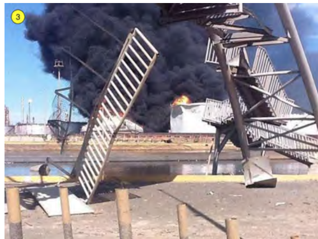
Figure-S 4.8 Close up of footbridge showing damaged railings and supports drawn towards the refinery. (Figure taken from [10].)
