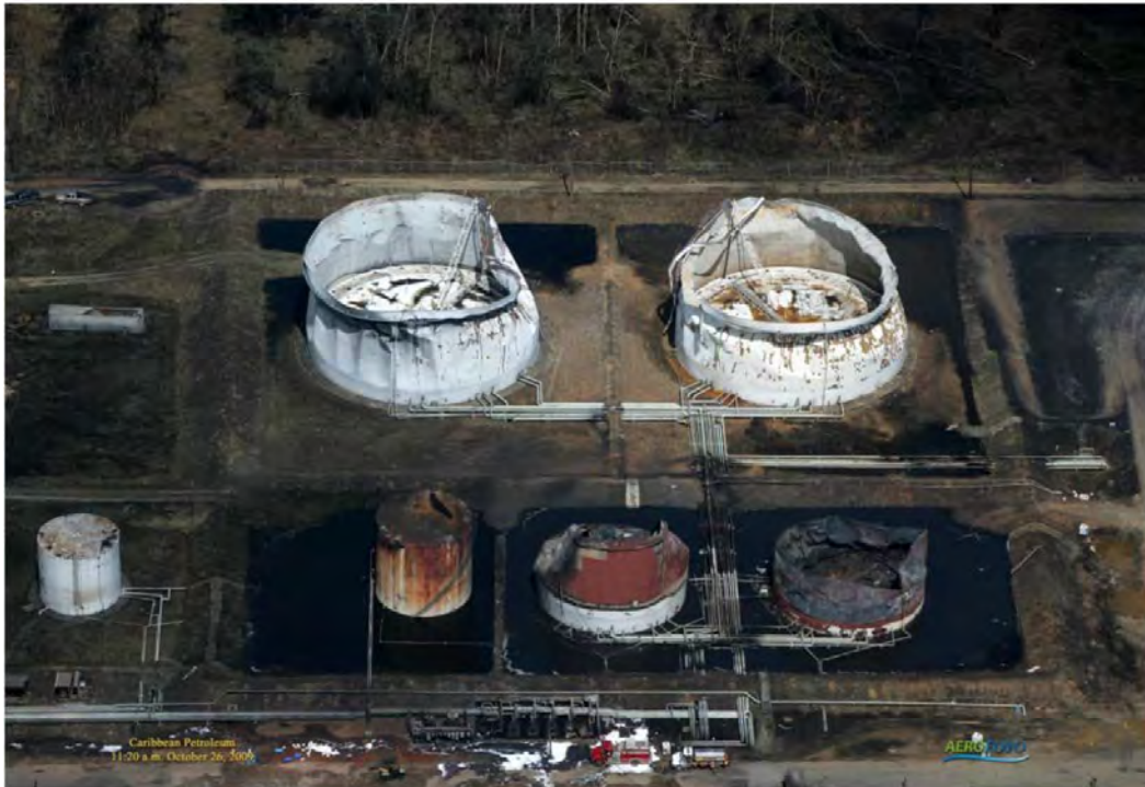
Figure-S 3.6 Blast damage to empty tanks 406 and 407. Figure Figure-S 3.3 was taken from left side of this figure [6].
