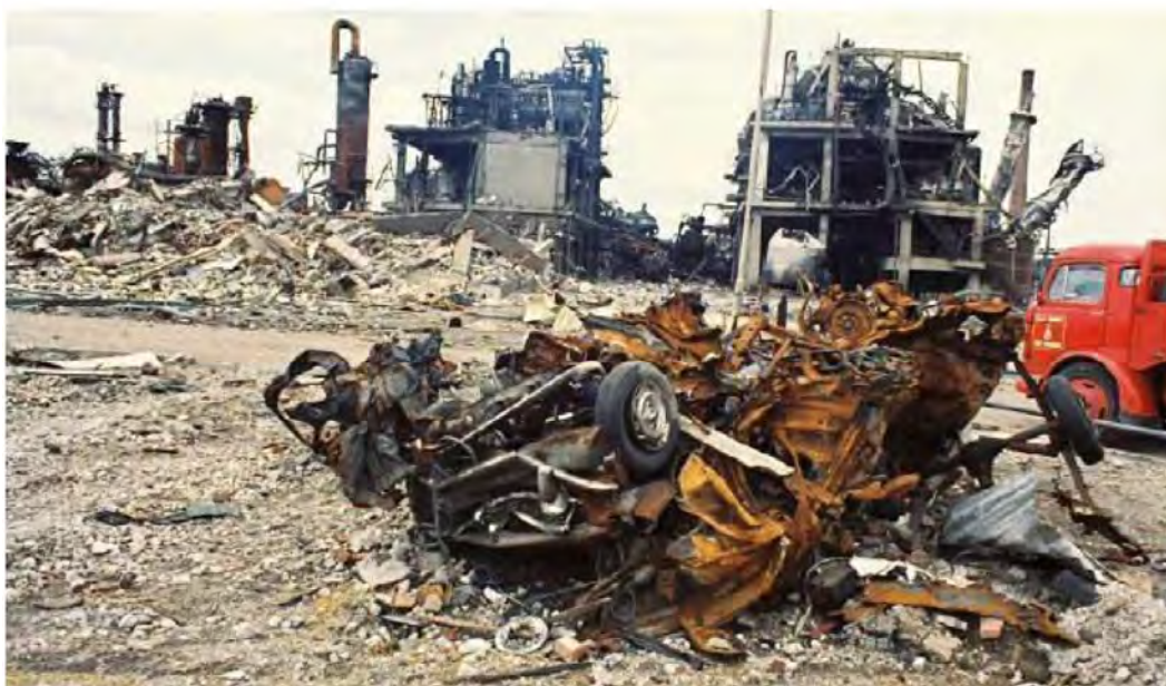
Figure-S 10.2 View of damaged items [23, 24].
