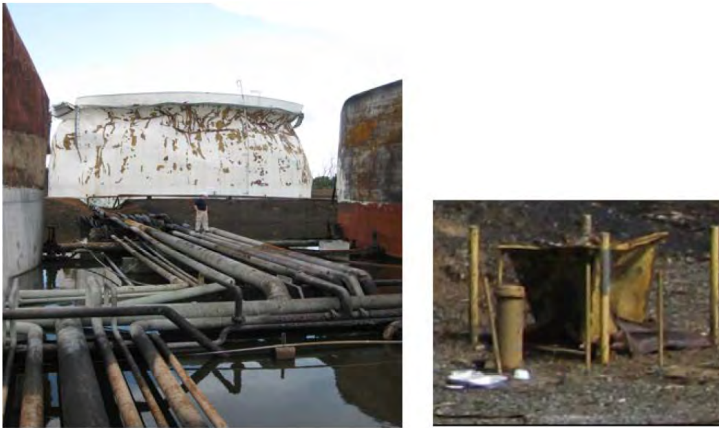
Figure-S 3.17 Congested pipework in the region between tanks 404 and 405 (triangulated area) (left) and crushed steel box (right) 70 m to the east of the triangulated region [6]. . Note uniformly crashed tank.
