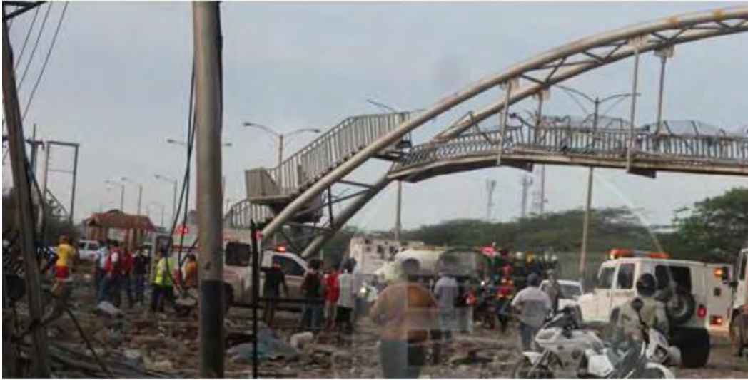
Figure-S 4.7 Note footbridge drawn inwards towards refinery, suggesting footbridge inside detonation. (Figure taken from [10].)
