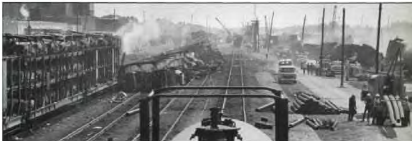
Figure-S 12.2 Damage area (taken from [26]).
