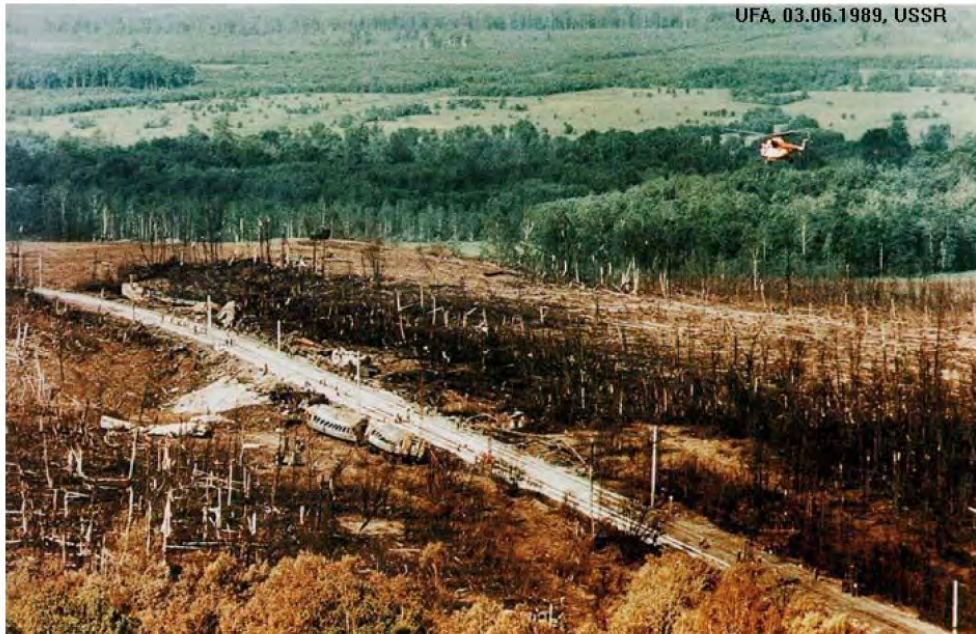
Figure-S 7.5 View after the accident. Note crushed train on left side (G.M. Makhviladze, private communication).
