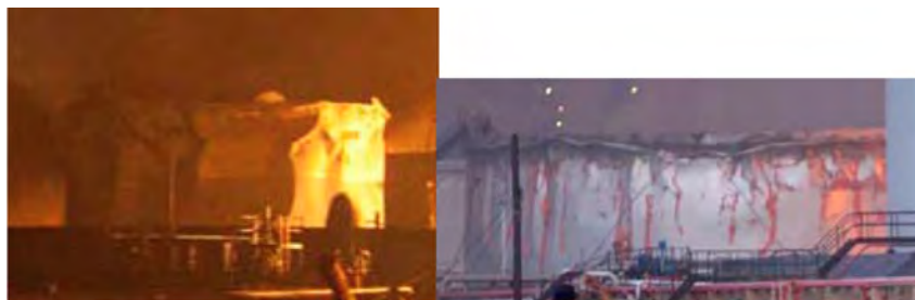
Figure-S 4.15 Crushed storage tank suggesting detonation impact. (From website Runrun.es, by permission [11].)
