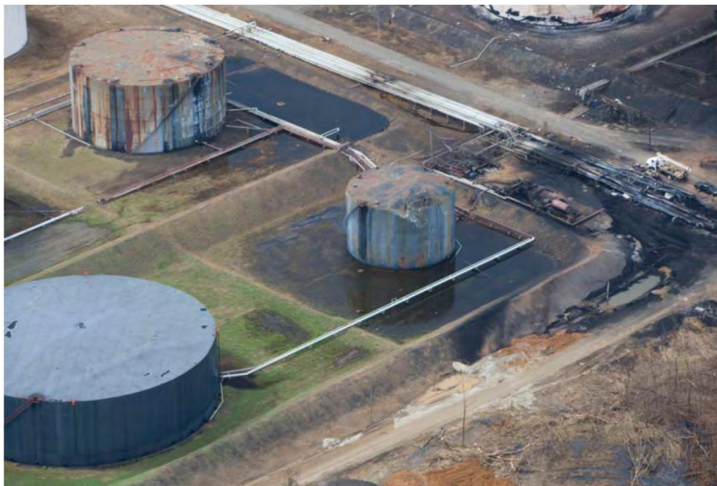
Figure-S 3.7 Tank 607 is the smaller tank near the center of the picture [6].
