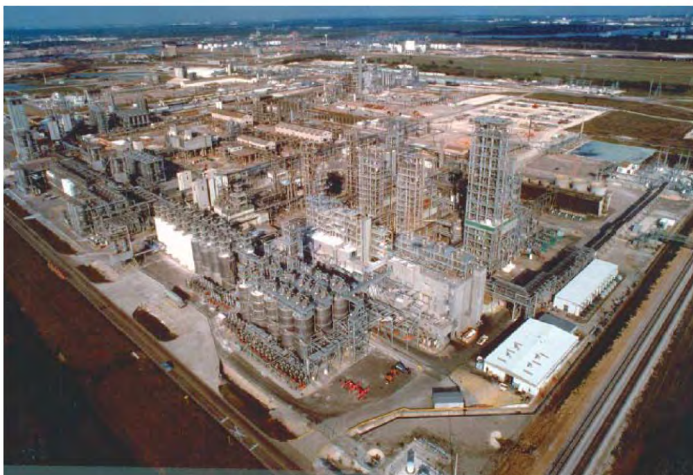
Figure-S 11.1 Aerial view of the Phillips plant taken prior to the explosion (taken from [25]).
