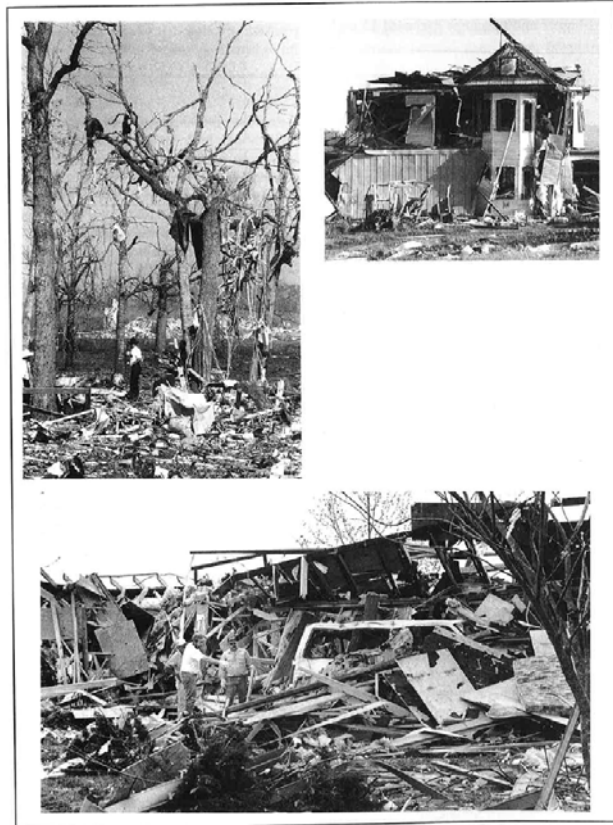
Figure-S 6.4 Area residences damaged by blasts. Sketch reproduced from [14]. Top right: a building about \sim 800 m from the release point.
