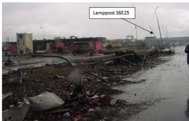
Figure-S 5.7 Panorama of the west side of Unit 40 south end, electrical building. Note the bent lampposts all drawn inwards, i.e. towards the centre of the flammable cloud. (Private communication to GAC, 2004).
