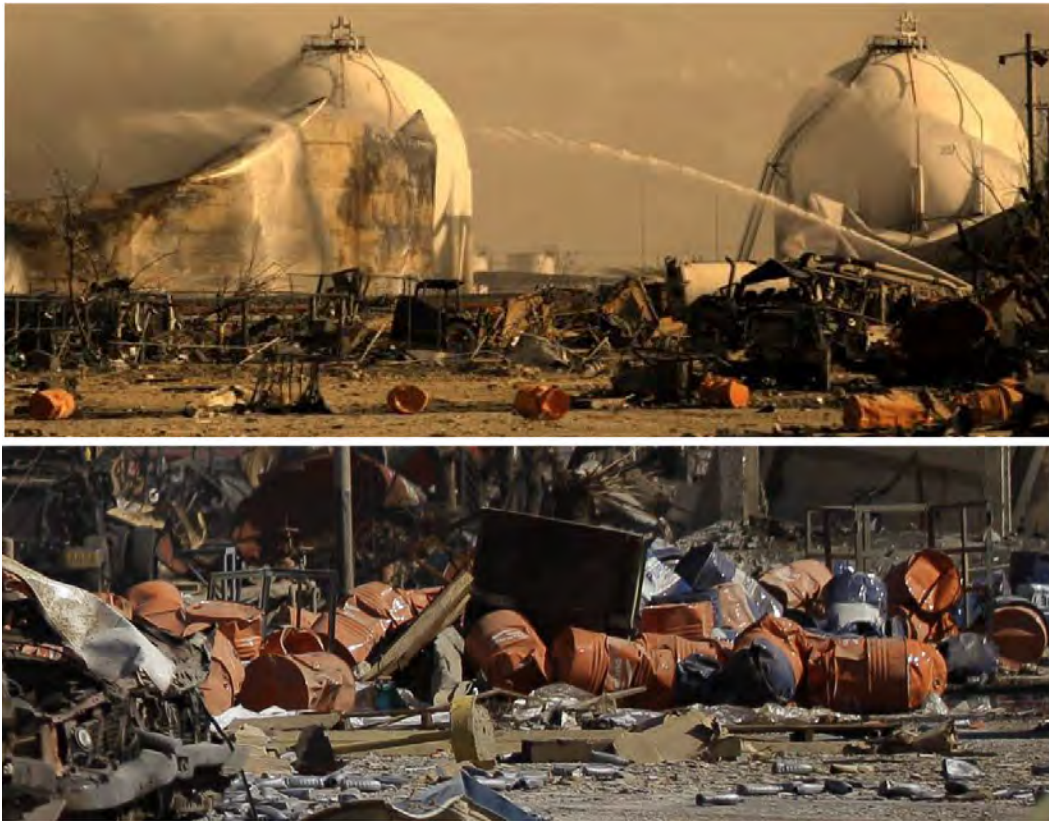
Figure-S 4.12 Top: Drums and car damage. Bottom: Enlargement of Figure-S 4.10 showing creased drums. (Figure from CTV News, August -September, 2012.)
