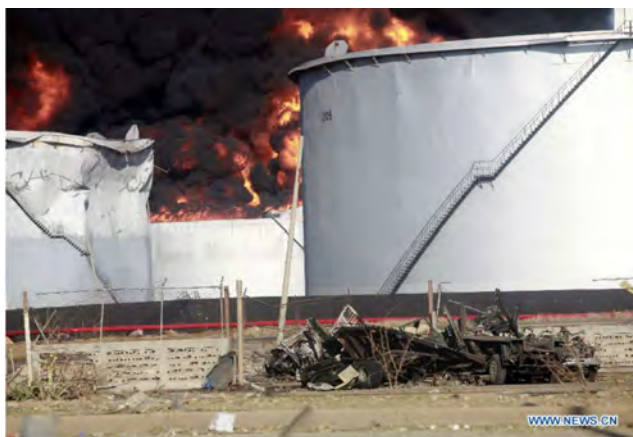
Figure-S 4.14 Crushed storage tank. Notice damaged cars.
