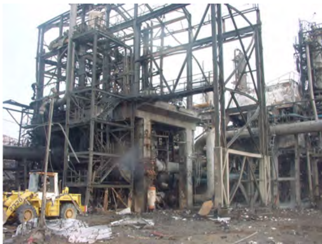
Figure-S 5.8 West side of Unit 40. Note that the tower by the yellow truck has been drawn
