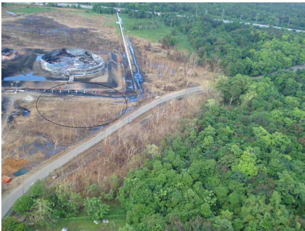
Figure-S 3.5 The damage to the area that once contained dense vegetation is shown inside the superimposed black oval ring in the middle of the left side of the photograph [6].
