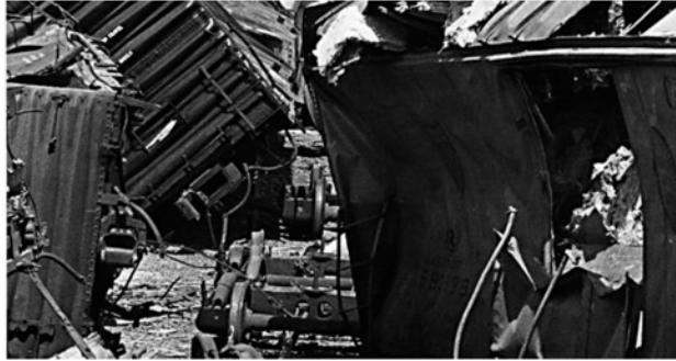
Figure-S 12.3 View of damaged items (taken from [26]).
