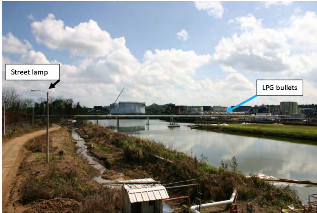
Figure-S 3.3 View from the waste water treatment CCTV camera (also called the NW camera). Note crushed white tank [6].
