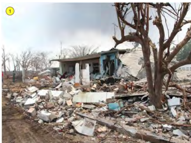
Figure-S 4.16 Building damage in the vicinity of the car allegedly responsible for ignition of the cloud [10].
