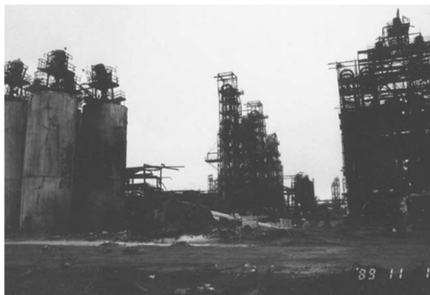
Figure-S 11.4 Silo holding areas to the northwest of the main blast area. The blast wave partially flatten the silo sides (taken from [25]).
