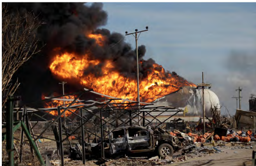
Figure-S 4.10 Lube oil plant damage to truck and oil drums. Note building destroyed, but poles not bent.
