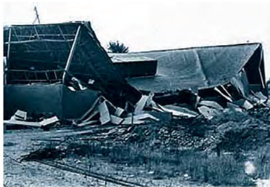
Figure-S 12.5 The explosion leveled the new school addition to the Lakeview High School building (taken from [26]).
