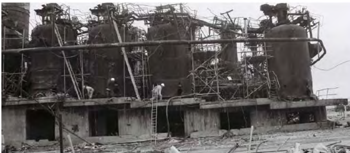
Figure-S 10.1 Photograph of part of the reactor train after the incident [23, 24]. The dog-leg bypass connecting the gap to the last vessel was lost completely. The scaffolding was been erected after the incident
