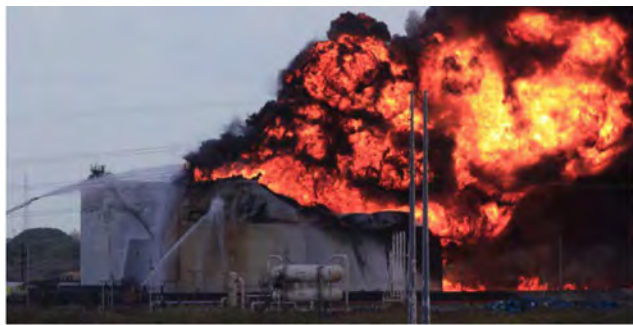
Figure-S 4.13 Crushed storage tank with tank top fire that melts and deforms the tank walls.
