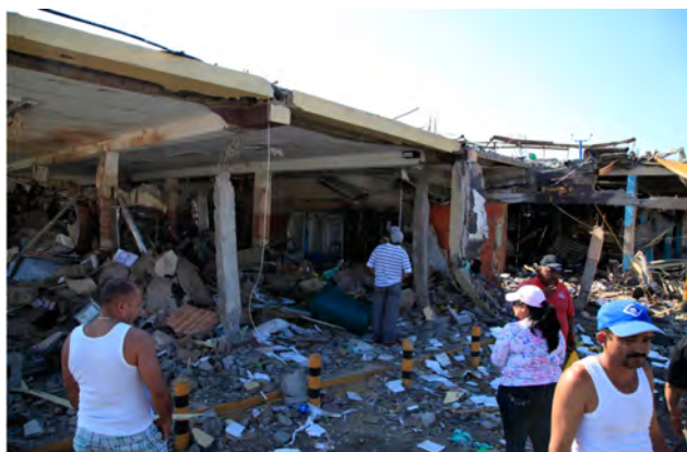
Figure-S 4.3 Houses adjacent to road running east of the lube oil area. Notice displacements of reinforced concrete poles. (Figure taken from [10].)
