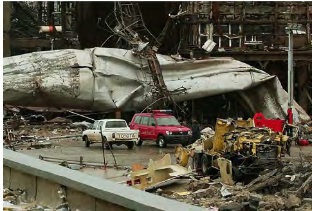
Figure-S 5.9 Unit 40 and the heavy duty car crushed; overpressure above 5 atm away from congestion. (Private communication to GAC, 2004).
