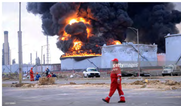
Figure-S 4.6 Crushed storage tanks. (Appeared on website of Christian Science Monitor , 16 September 2013. )
