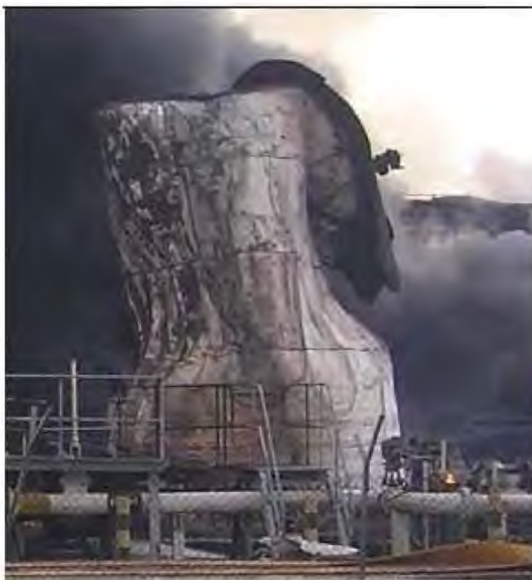
Figure 4.7 Crushing damage to partially empty tank 601 at Buncefield [48].
