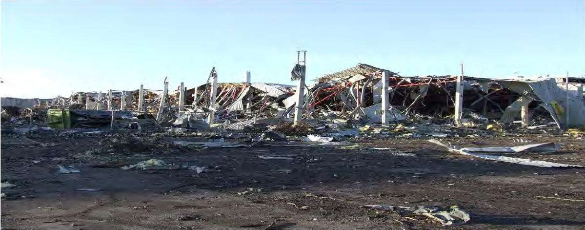
Figure 5.1 The destroyed south side of the Fuji Building at Buncefield. The building was on the west side of an open car park [3].
