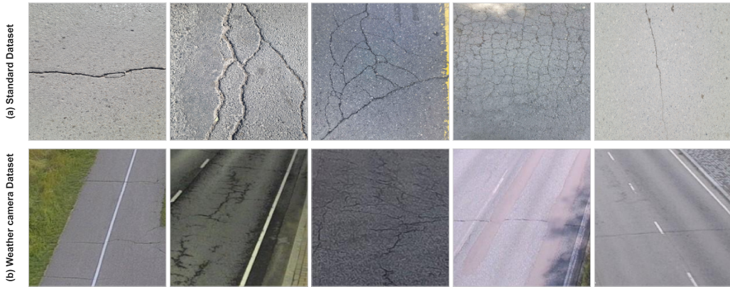
Figure 10 Illustration of the domain shift between datasets. (a) The source domain (Standard Dataset) containing high-fidelity crack samples. (b) The target domain (Weather Camera Dataset).
