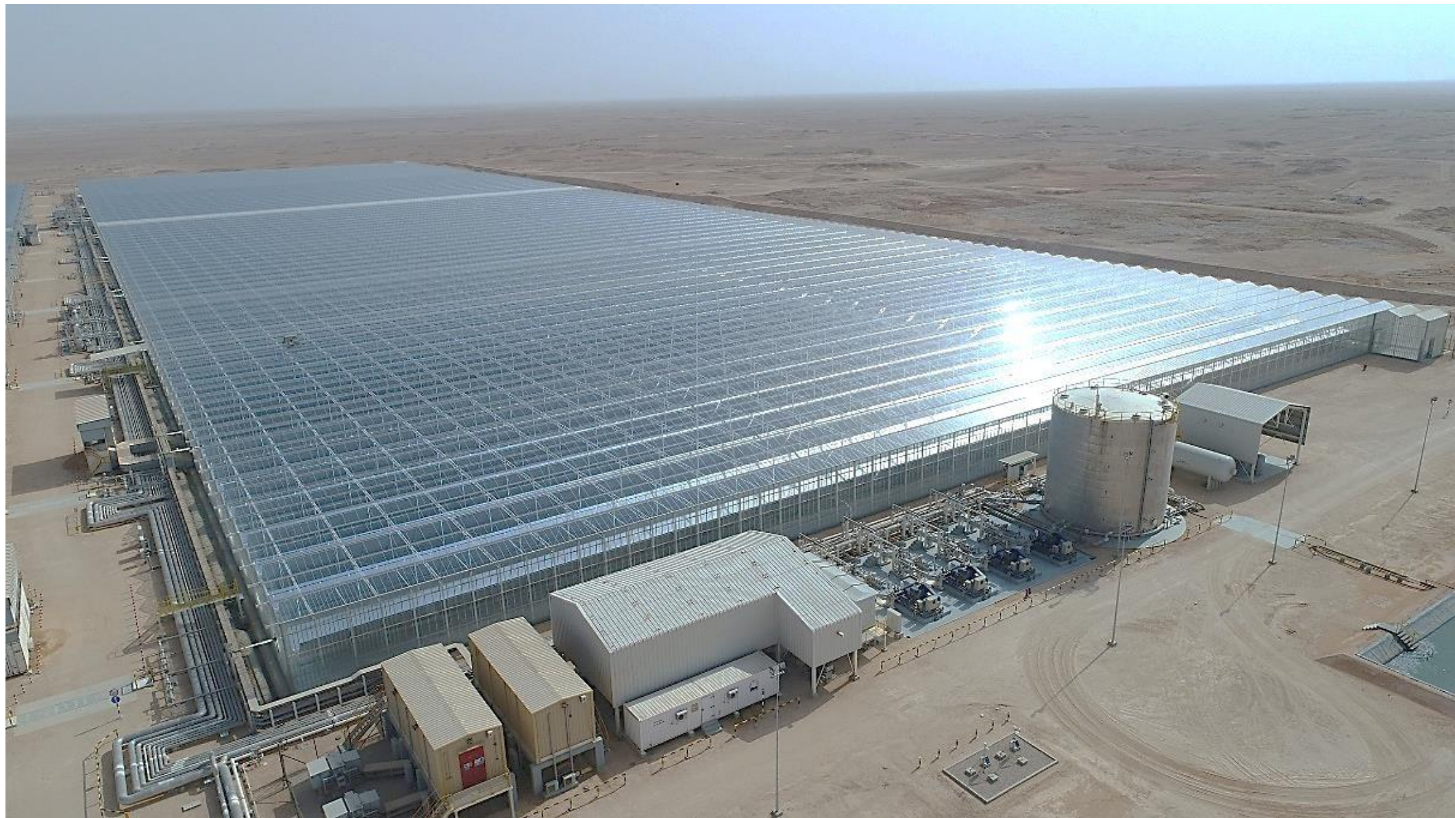
Fig. 5. photograph for the HEOR system “Miraah” (© GlassPoint, reproduced with permission)
