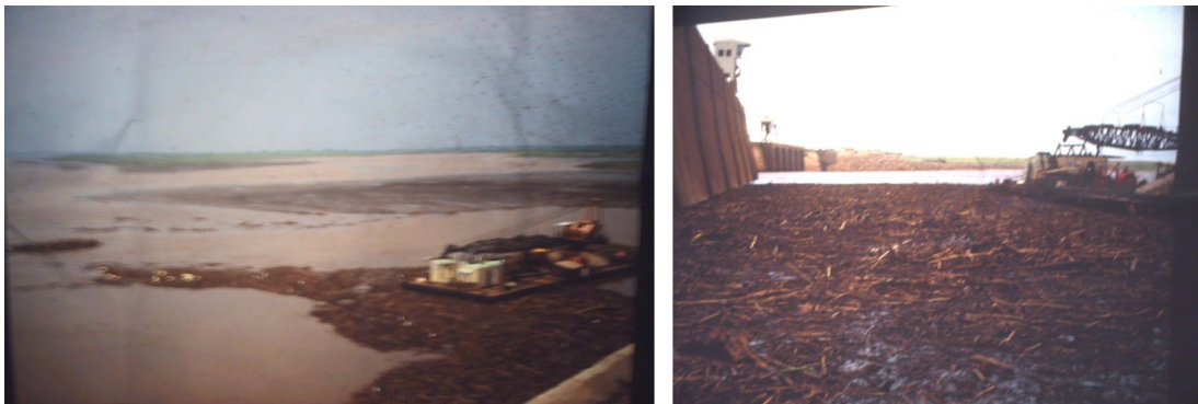
Plate (1) Delta Formation Upstream, Roseires Dam (left) | Plate (2) Debris in the Reservoir Upstream, Roseires Dam (right)
