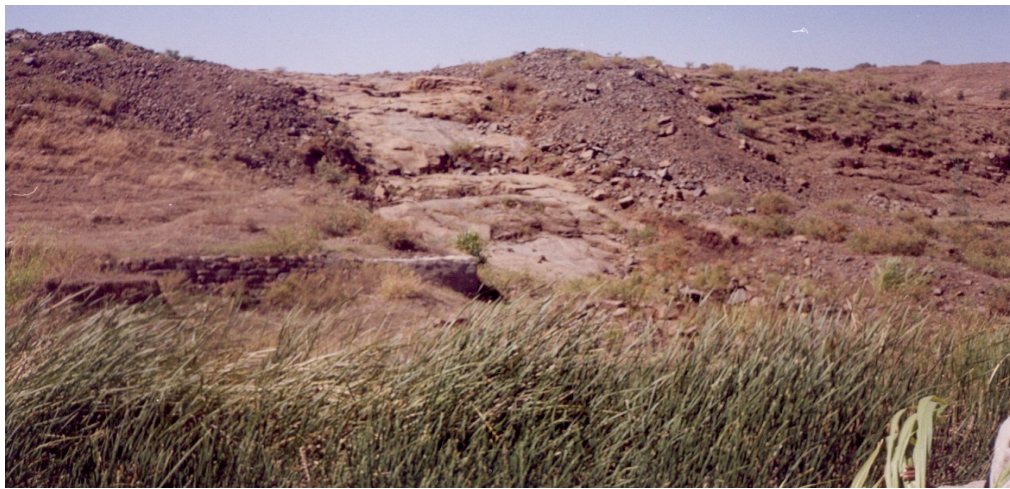
Figure 4.3 Photograph Showing Part of Spillway
