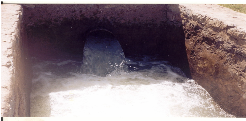
Figure 4.4 Photograph Showing the Irrigation Outlet
