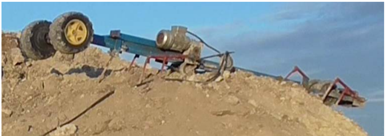
Fig. 11: After a few more centimeters of extension and thanks to the extra ballast the front end becomes too heavy. UTOPUS swings over the edge such that the front crampons can engage the soil.
