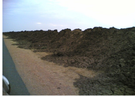
Plate 2. Accumulation of Sediment on Canal Banks
