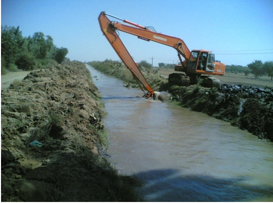
Plate 1. Canal Sediment Clearance
