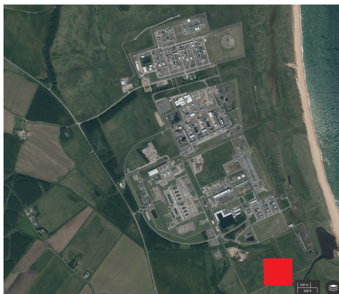
Figure 15: Overhead photograph of the St. Fergus gas processing plant. The red square represents the size of the required 50MW e /100MW e powerplant relative to the site.
