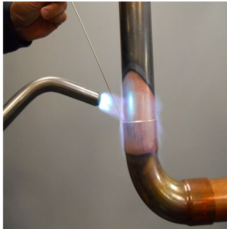
Figure 6.1: Brazing process
