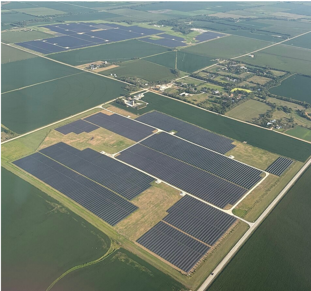
Figure 4.1 Aerial view of a ground-mounted photovoltaic installation near Mead, Nebraska, USA. Photo: AllTheUsernamesAreInUse, Wikimedia Commons, CC0 1.0. Source: Wikimedia Commons. Available from: https://commons.wikimedia.org/wiki/File:Mead,_Nebraska_solar_farm_aerial_2026_(cropped).jpg
