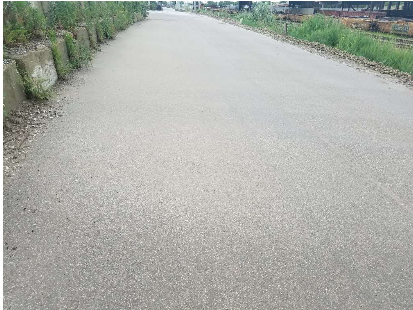
416 417 Fig. 4 Surface condition of Pulaski test site in July 2017, after 3 years of service.
