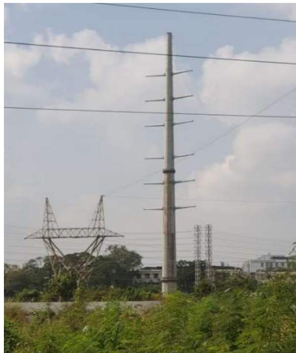
Figure 2 Pipe Section Transmission Tower Profile
